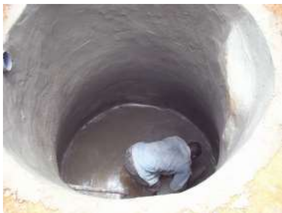
Regenwassertank in Mmuock, 2009
